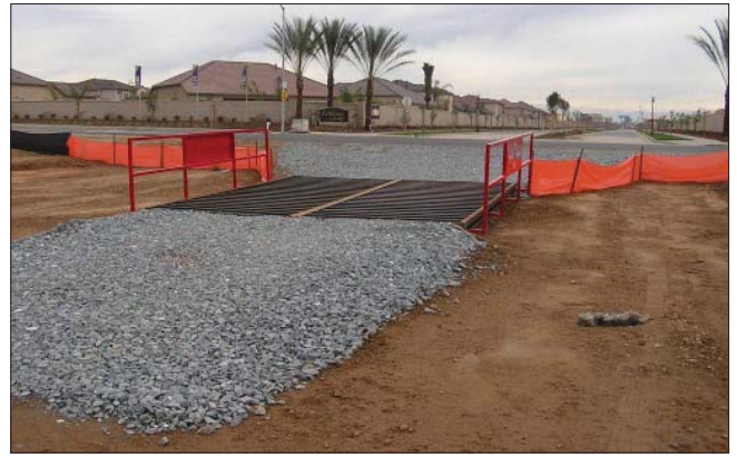
Well-developed trackout control using rock, rumble strips, and silt fences.
