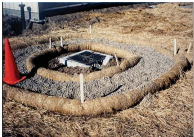
Protecting an interior drainage inlet.
