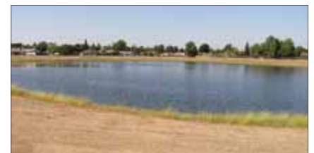
One of more than 80 District basins used for artificial groundwater recharge.
