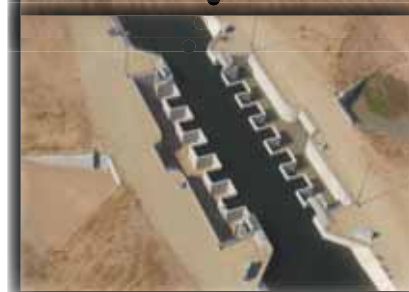
PLEATED WEIRS - Allow flood water to be moved from the channel to the two large detention basins on either side. Together, the basins have the capacity to hold 1,890 acre-feet of stormwater.
