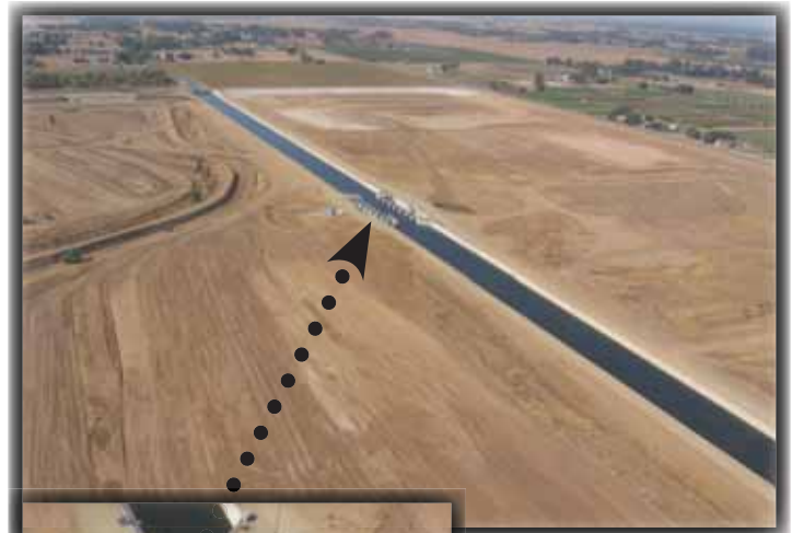
PLEATED WEIRS - Allow flood water to be moved from the channel to the two large detention basins on either side. Together, the basins have the capacity to hold 1,890 acre-feet of stormwater.
