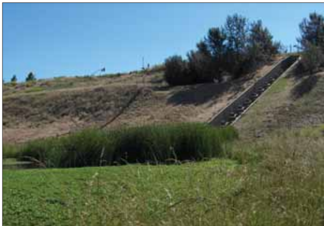
Storm drainage channel serving a neighborhood just south of the river delivers water to the created wetland along the MacMichael Trail, near the Jensen River Ranch.
